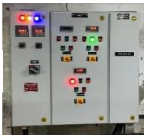
Lift Pump Electric Panel
