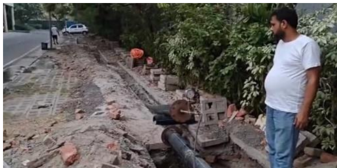
HDD Trenchless Work in Progress
